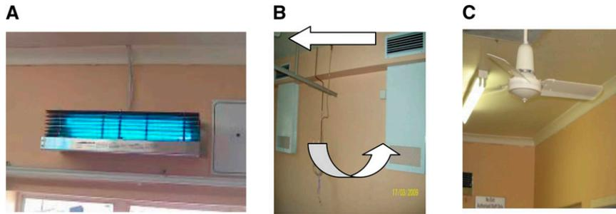
**Figure 2.** (A) Ultraviolet germicidal irradiation wall fixture, (B) room ventilation arrangement, and (C) ceiling paddle fan model in use during experiments. Note that the photograph in A was taken wearing ultraviolet protective goggles because even brief direct exposure at close range to upper room ultraviolet germicidal irradiation lamps can cause corneal inflammation. The arrows in B indicate air movement.
